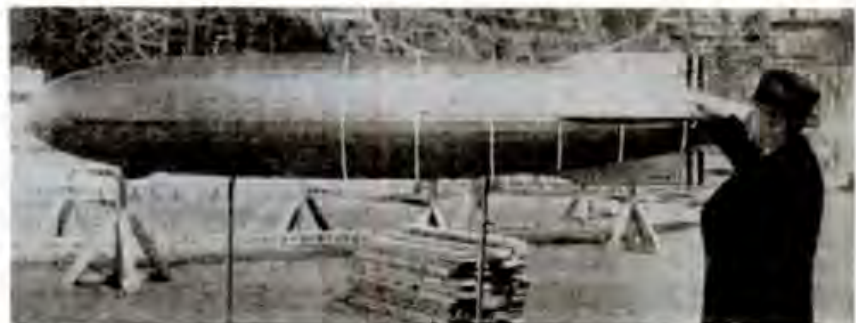
Here is a scale model of the "Macon," showing how it will appear when completed. Standing beside it is Dr. Carl Arnstein, the designer of the Akron and the Macon.
